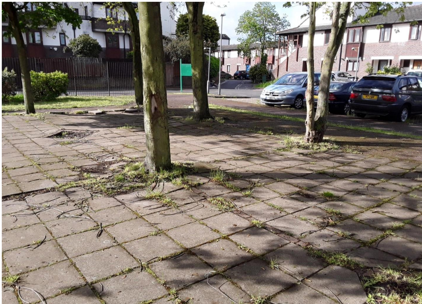
Figure 3 The existing paving slabs and hardstanding that surround the trees (to be removed).
