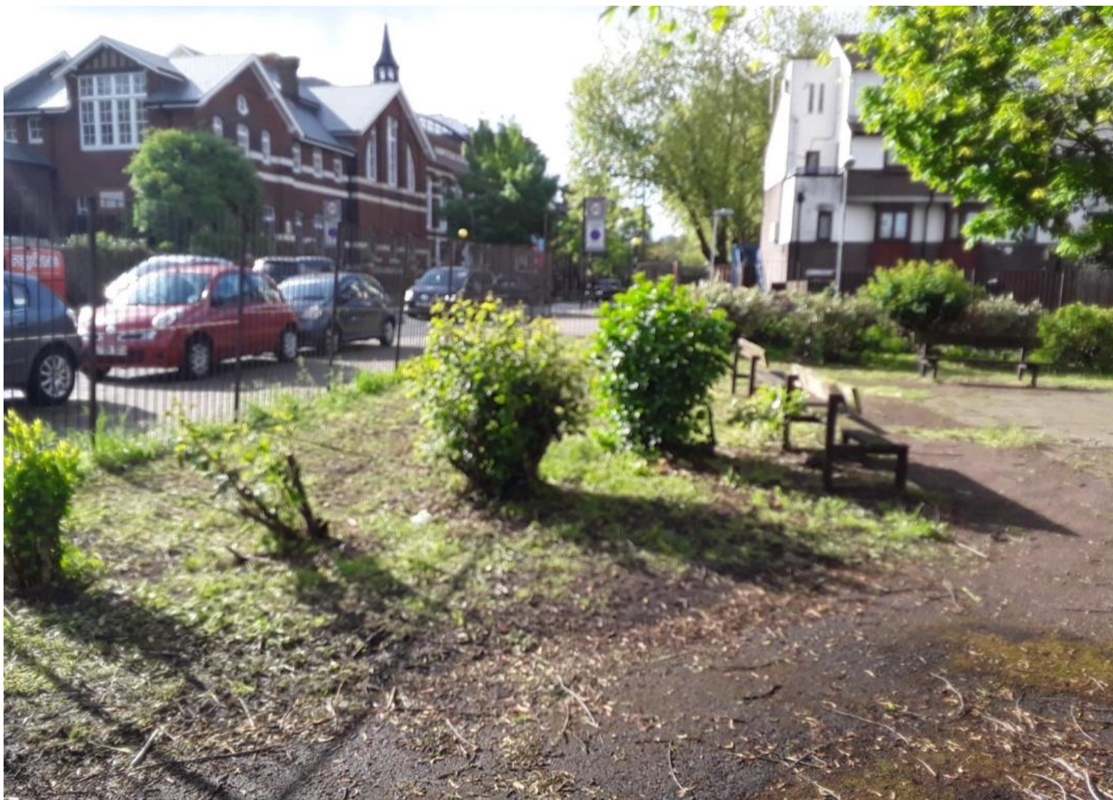
Figure 5 Tarmac to be removed
